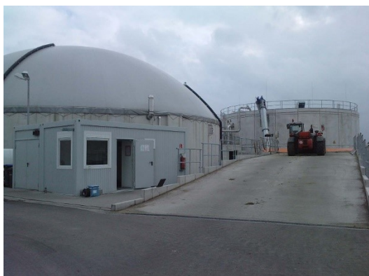
Picture: DSM Biogas
